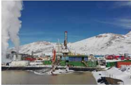
RIG H202. Cerro Pabellón, Chile
